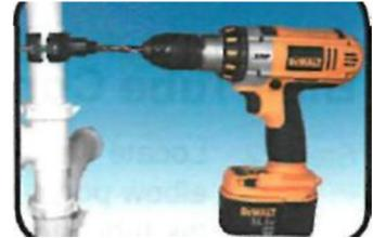
**Caution:** It is very important to keep the drill centered to prevent damage of the drain saddle while drilling.
