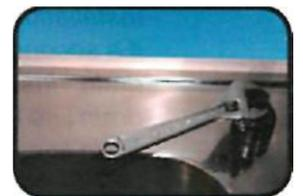
1/2" & 1 1/4" Hole Punch. The opening should be centered between the back splash and the edge of the sink, ideally on the same side as the vertical drain pipe.
